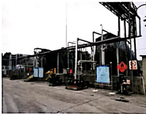
罐区 1 围堰 (730cm*650cm*105cm=49.8225m 3 )
