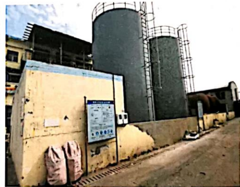
罐区 1 围堰 (730cm*650cm*105cm=49.8225m 3 )
